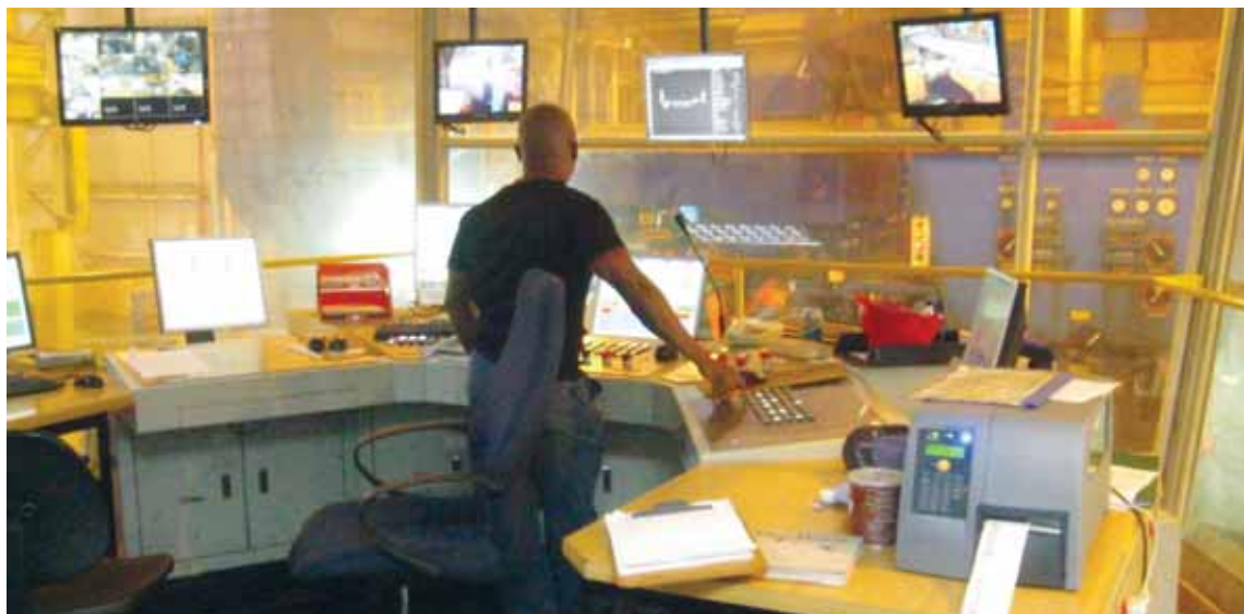
Figure 4. Double glazed control room
